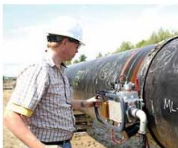
Weldstar mobile ultrasonic inspection system
